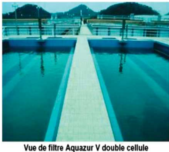
Fig. 6. Filters of 12 batteries.
