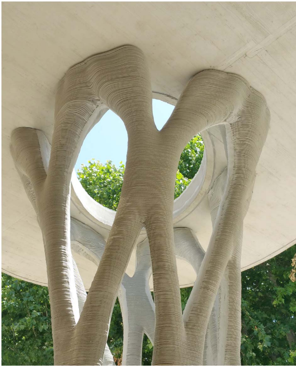
Fig. 4. Printed pillar in Aix-en-Provence (XtreeE, 2016).
