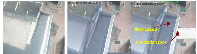
Figure 6: A) video of the building from UAV; B) superimposition of the video and BIM as a mixed-reality; C) annotation mode
