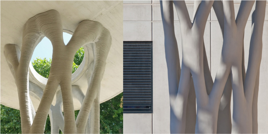
Fig. 11. Before (left) and after (right, photo by Lisa Ricciotti) surface smoothing through manual coating.
