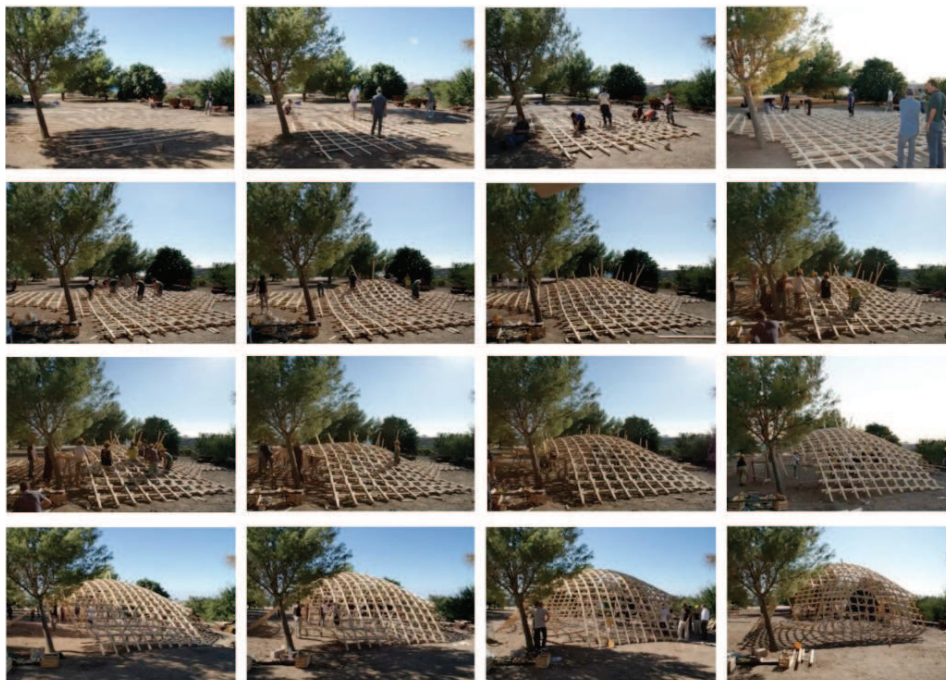
Fig. 2 Shaping process.
