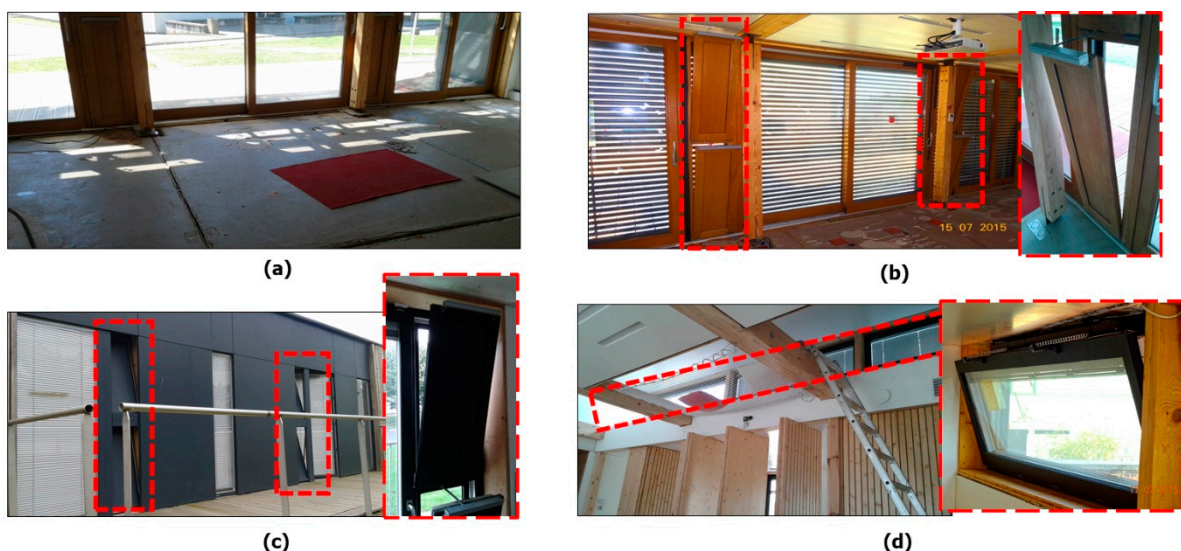
Figure 1. Architectural features: (a) floor concrete slab, (b) programmable solar shades and natural ventilation openings (inside red squares) on the south glazed façade, (c) the north facade, (d) and the shed roof.
