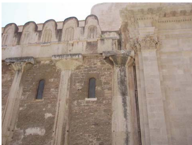
Fig. 1 Left side of the Syracuse dome (Italy). Columns of the Doric temple of V century AC were included in the wall
