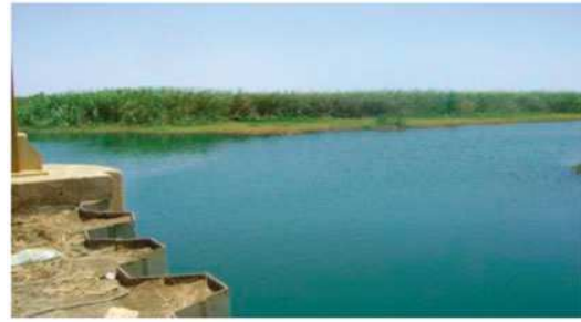
Fig. 3. The water intake from Aftout Es Saheli.
