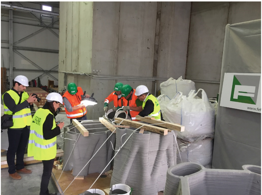
Fig. 9. UHPC casting inside the envelope, with supports left in place.
