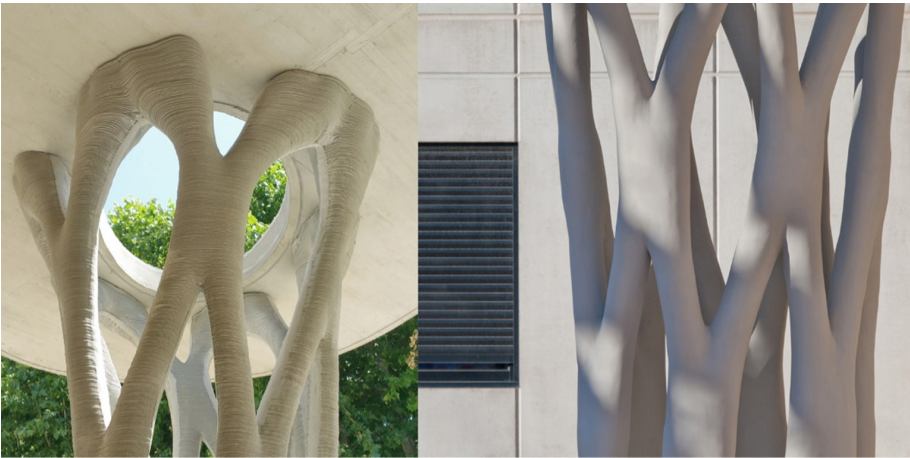
Fig. 11. Before (left) and after (right, photo by Lisa Ricciotti) surface smoothing through manual coating.
