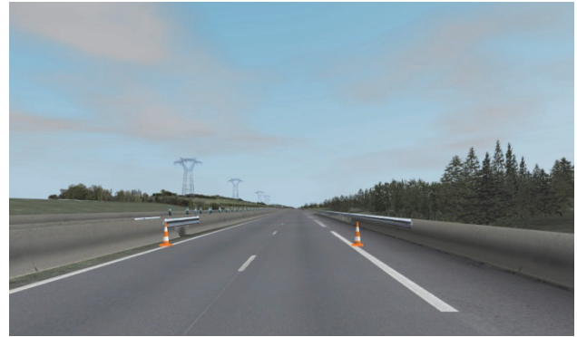
Fig. 4. Screenshot of the double-lane motorway.
