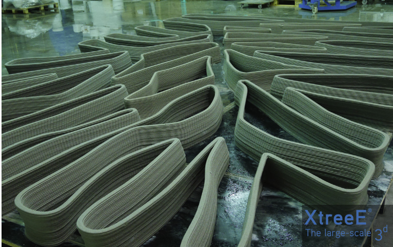
Figure 3.15 3D-printed concrete formwork for the YRYS Concept house interior wall.
