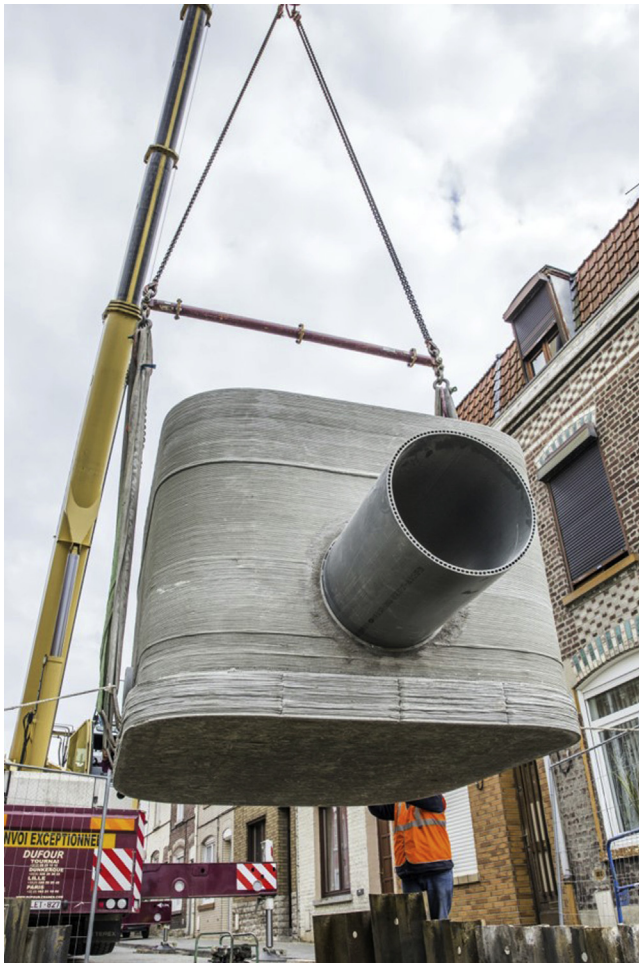
Figure 3.18 On-site lifting and placing operations for the rain collector.
