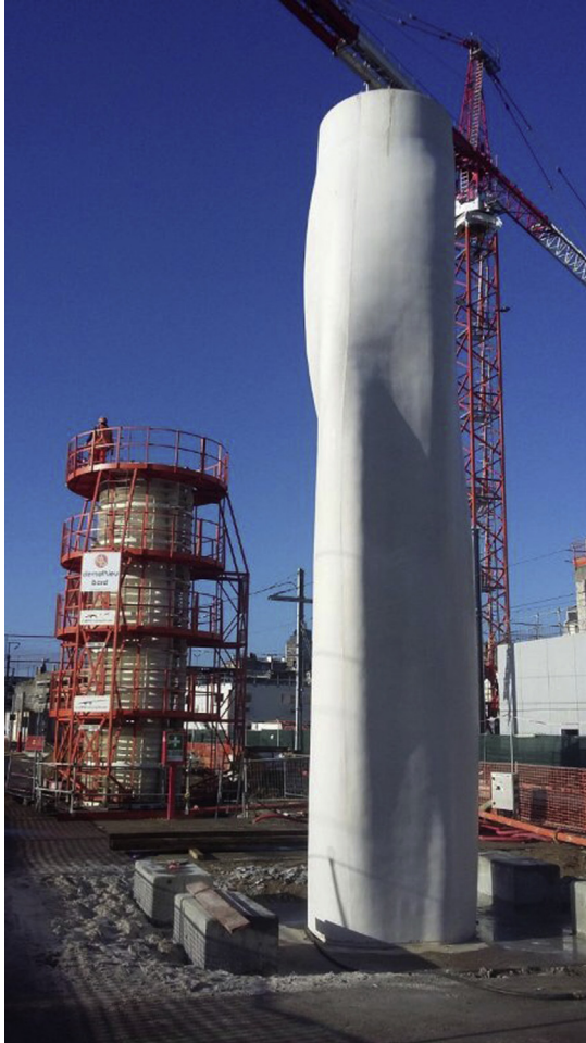
Figure 3.11 Example of semistandard shaped pillar on the construction site of the new train station of Nantes, France.
