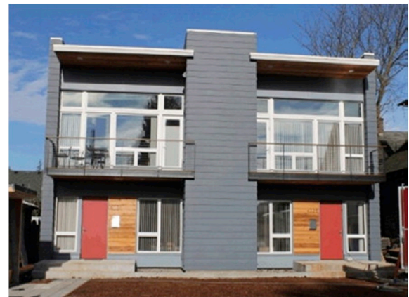
Fig. 15. The passive house duplex home [123]. Copyright (2019), with permission from Elsevier.
